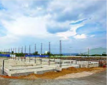
The Sanmenxia Power Generation Company's under-construction stand-alone shared energy storage station in the Sanmenxia Demonstration Zone has an initial capacity of 100 MW/200 MWh
