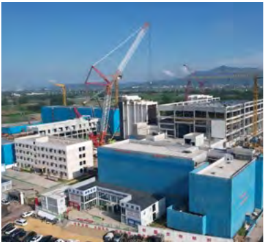
Boluo 2×460 MW gas-fired thermal power project
