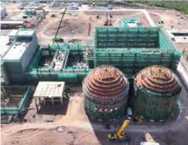
Ningxia Branch ramps up efforts and accelerates the construction of the Zhongning 100 MW/400 MWh compressed air energy storage project
